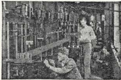
A Real Switchboard in the Coyne Shops
